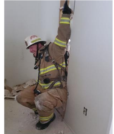
Interior Wall Breach Demonstration
