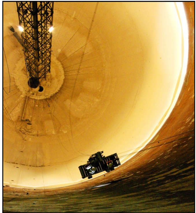
Navy-contracted workers inspect the wall of Tank 5 at Red Hill.
